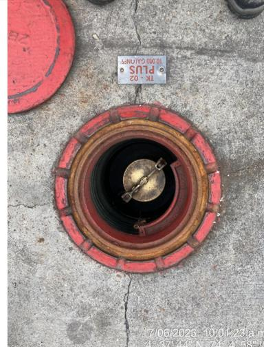
Foto 14. Spill-container tanque 2
