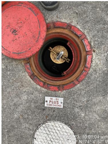
Foto 13. Spill-container tanque 1
