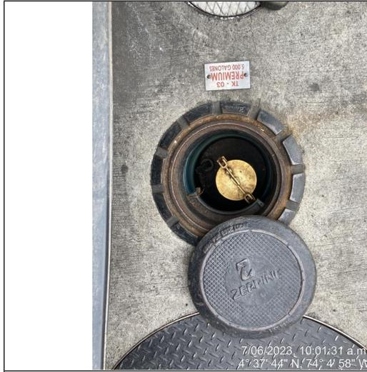
Foto 15. Spill-container tanque 3 -1
